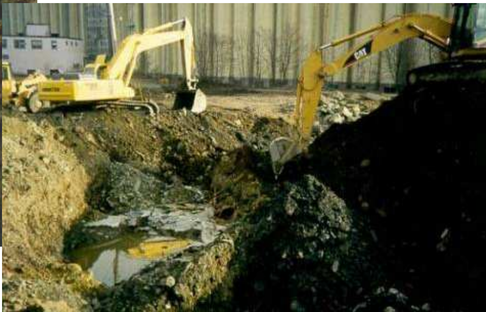
1997-1998: Site Remediation (Dig and Truck)
